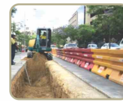
UNDER GROUND ELECTRIFICATION
